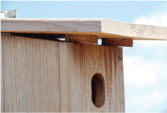
Roof front lifted and blocked for venting
